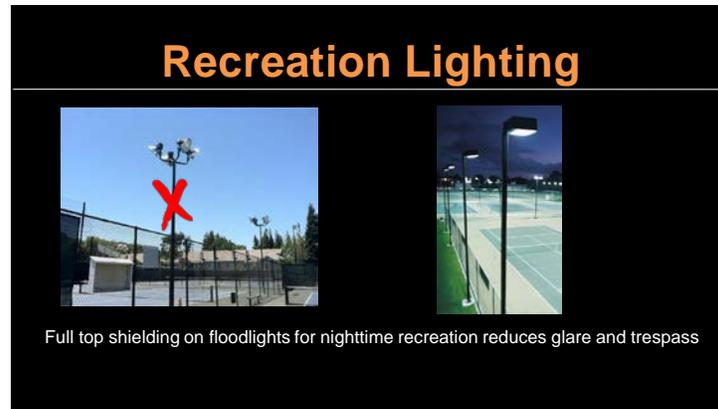
When a recreation use require floodlights for night activity, full cut-off is highly recommended, such as the example on the right. The left is not fully shielded and is angled upward, which can cause glare and trespass.
