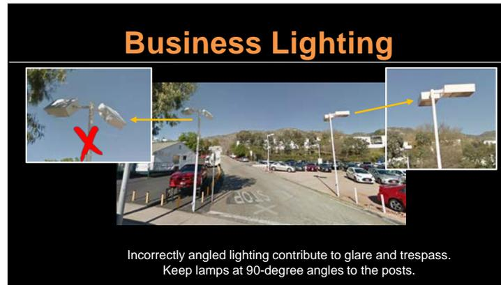
Here is an example of angled lighting in a parking lot - the post on the left is incorrectly angled sideways which cast glare across the entire parking lot and may spill over to the street or adjacent properties depending on how it is angled. The lamp on post on the right is correctly angled downward at 90 degree-angles.
